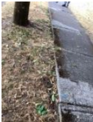
Hazard # 52 7940 Lake Forest Dr SE CAN SEE BOTTOM OF PANEL, NOT ENOUGH PANEL TO CUT
